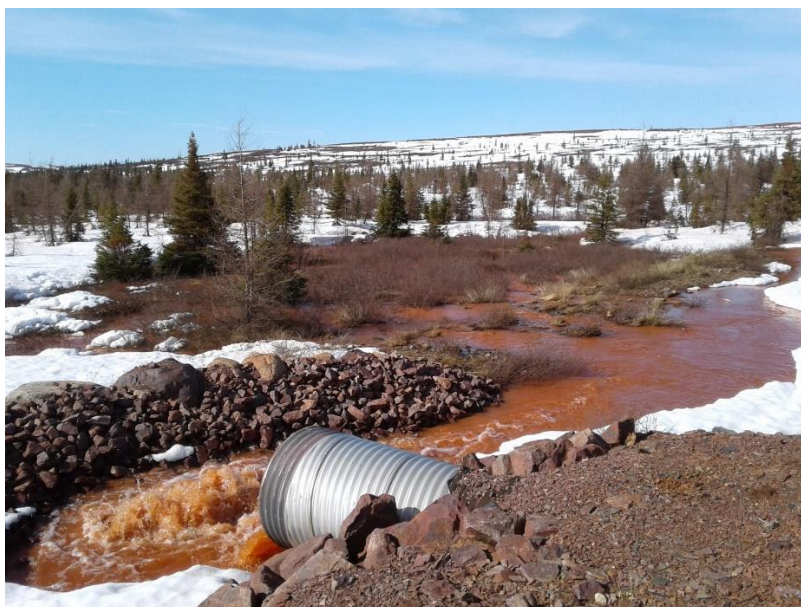
Figure 4. Water flowing from culvert into adjacent wetland.
