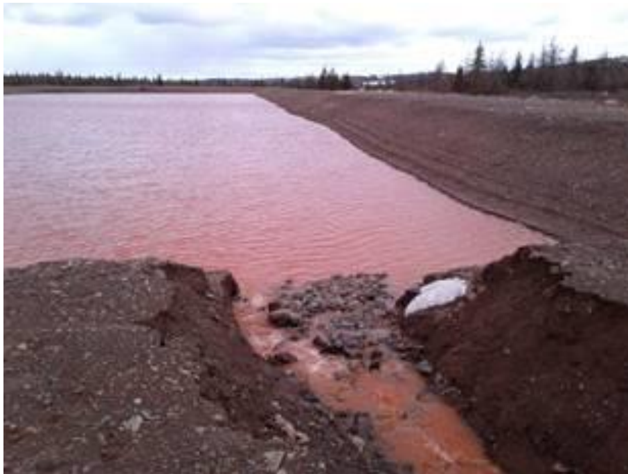
Figure 9. Low flow into breach prior to TSMC intervention.
