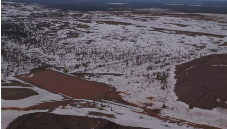
Figure 5. Aerial view of SP3 and associated infrastructure.
